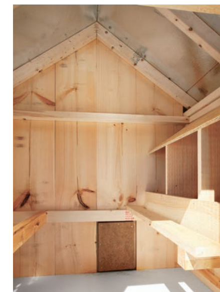
Interior view - A46
