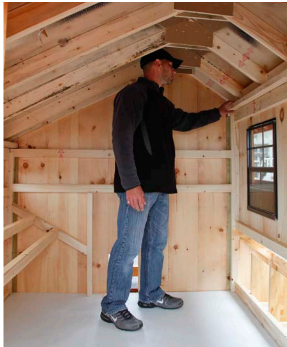
Interior view of Q612C (pages 30-31)
