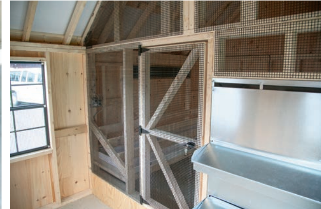
Screened wall with screened door
