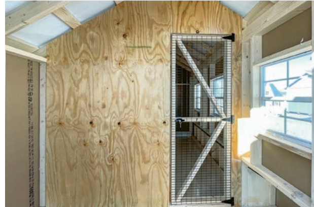
Solid plywood wall with screened door
